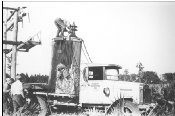
Dangerous work with some serious high voltage.
