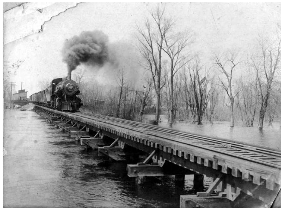
The Monon Trestle - Roselawn
