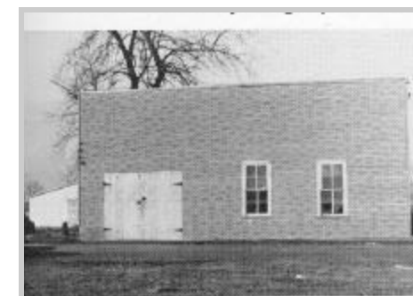
This photo also from "The History of Newton County, 1985", is the building in which a blacksmith shop owned originally by George Corbin was located. Later Eli Chupp, who worked for Mr. Corbin, took over the business. Ca 1908-1910.
