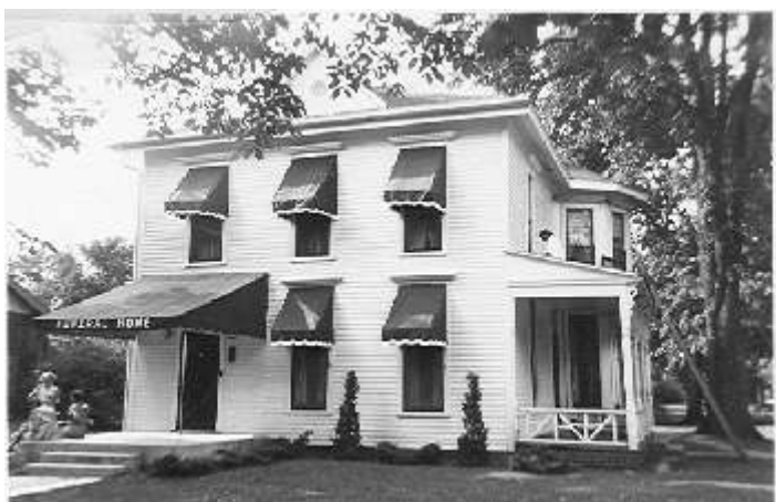
Hufty-Crane Funeral Home.
