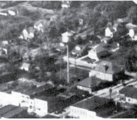
Morocco's water tower was erected with the help of PWA and WPA programs in 1938. This photo taken in 1951 shows a different tower than the one that stands today.
