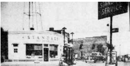
B.E. Childress Service Station, located at Hwy. 24 and 3rd Street since 1936. The new station was built that year in July, owned by Blanchard and Mary Childress.
