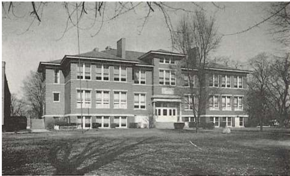
This picture shows the 1913 building with the door to the cafeteria and the east edge of the new gym.
