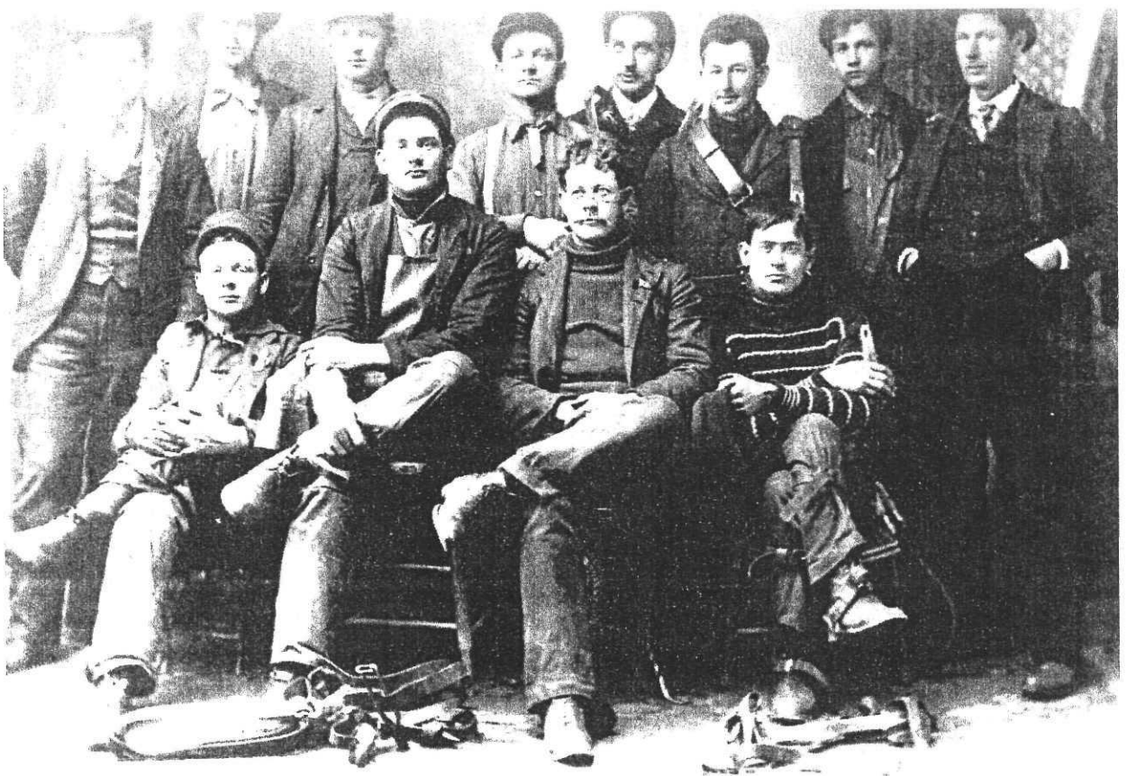
Princeton Telephone Company Construction Crew, March 17, 1902
